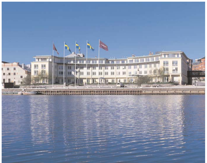
AstraZeneca's R&D center at Södertälje, Sweden, has some 35 video systems
